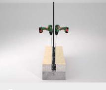
Perforate the slab with the drill, place the profile, fixing screws
